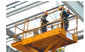
Aerial work platform at construction site
